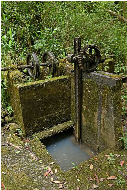
Fig. 13. Station 6b. Active Wailua Ditch intake W-18 along Hanehoi Stream.
