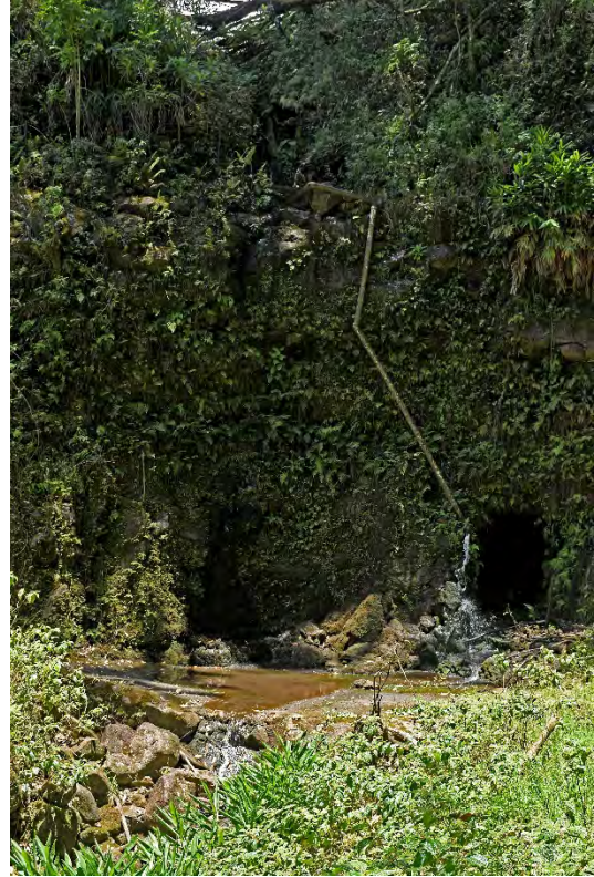
Fig. 25. Station 10, tributary to East Wailuanui Stream at Koolau Ditch intake K-20a.
