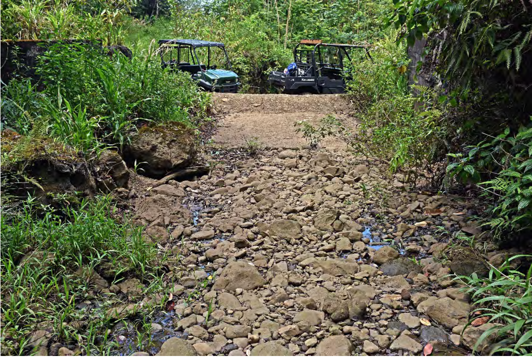
Fig. 15. Station 6a, Hanehoi Stream looking downstream to New Hamakua Ditch intake NH-17. The stream channel is nearly dry downstream of the concrete weir. All diversion at this site is being accomplished via the Wailoa Ditch intake W-18 further upstream.
