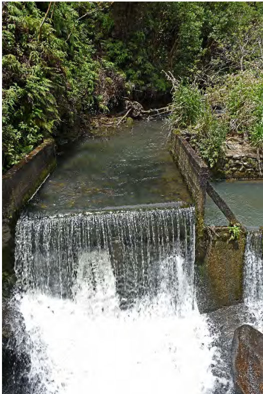
Fig. 5. Station 3. West Hoolawanui Stream tributary looking upstream at New Hamakua intake NH-20.
