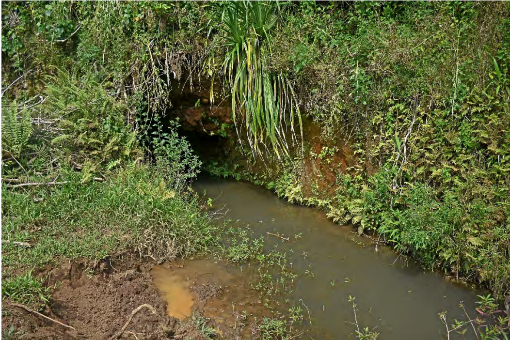
Fig. 18. Station 2, Lowrie Ditch and associated tunnel a short distance east of the Long Strainer and intake L-15.
